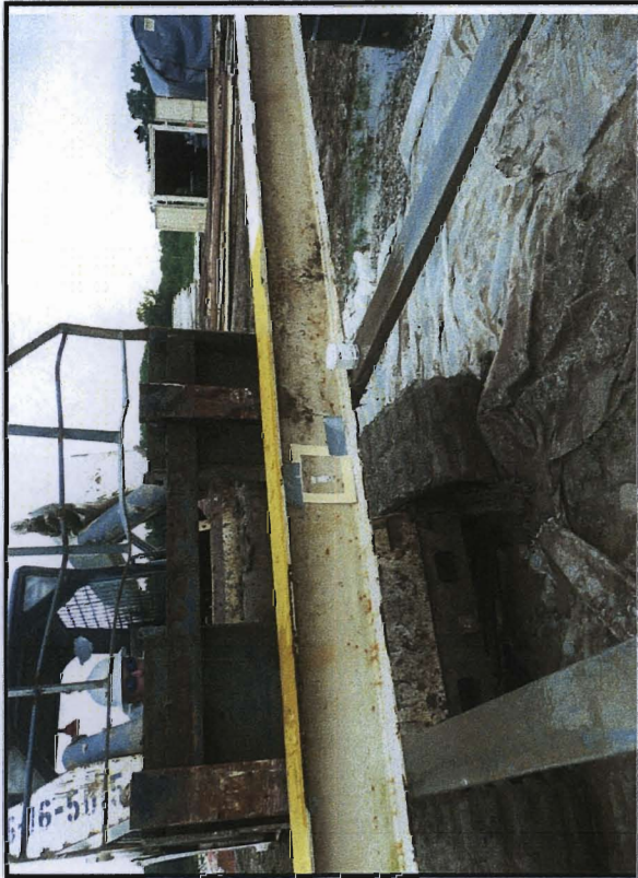
Photograph 55 | Wipe Sample Location # 709T23
